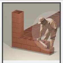
Place dry elements of the fence by pushing the blocks together; The blocks should be placed tight to each other. Check the horizontal and vertical before placing each layer. Minimize any horizontal deviation by grinding or using nog.
